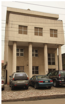
Front facade of Center for Contemporary Art, Lagos. Photo by Richard McCoy
